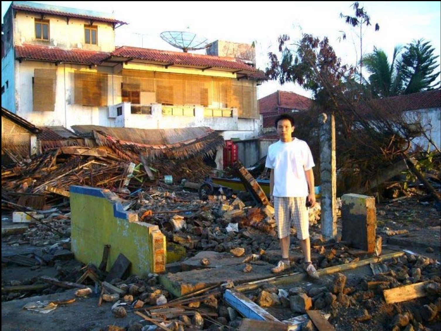
Pangandaran. Walls perpendicular to wave are often knocked down and walls parallel remain.
