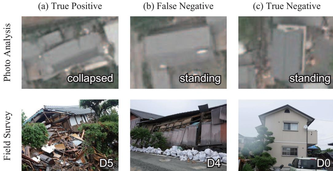
**Figure 15.** Examples of the (a) true positive, (b) false negative, and (c) true negative of the damage level from the photo analysis and field survey.
