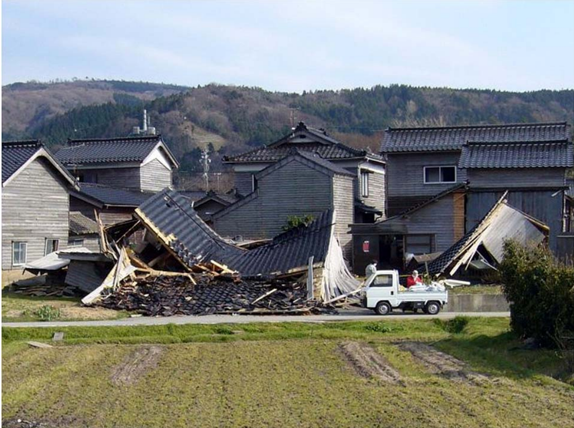
Figure 4: A totally collapsed house (Rank C).
