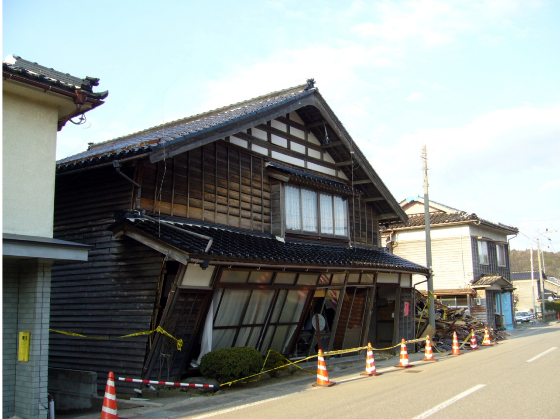
Figure 3: A house with severe damage on columns (Rank C). The columns are tilting forward more than 20 deg. and still standing.
