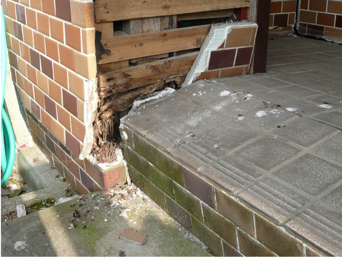
Figure 6: Termite damage on columns.
