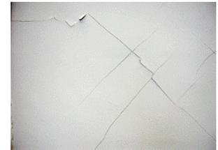
Photo 5. Cracks on a mud wall
