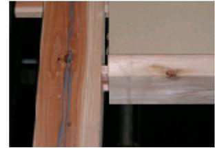
Photo 3. Separation of a lintel from a column
