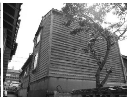
Photo 2 OUD Storehouse in Kuroshima (viewed from the sea side)
