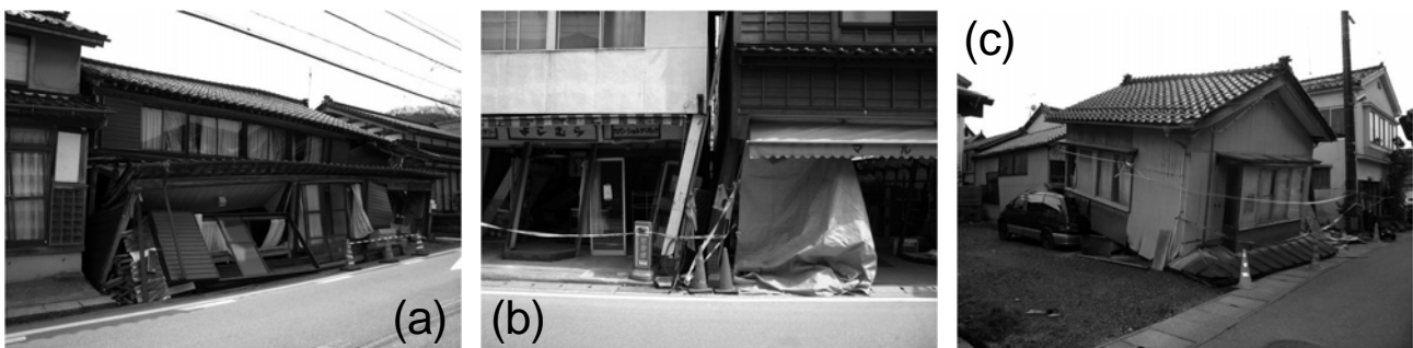
Photo 1. Examples of damage to wooden houses in (a), (b) Hashiride and (c) Anamizu during main shock.
