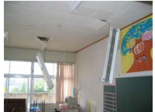
Earthquake damage at Kitamura Elementary School during the 2003 North Miyagi Earthquake, Japan
