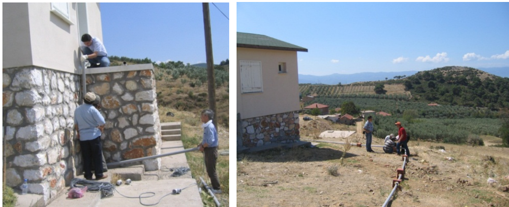
Figure 6. Construction of the IZN observatory.
